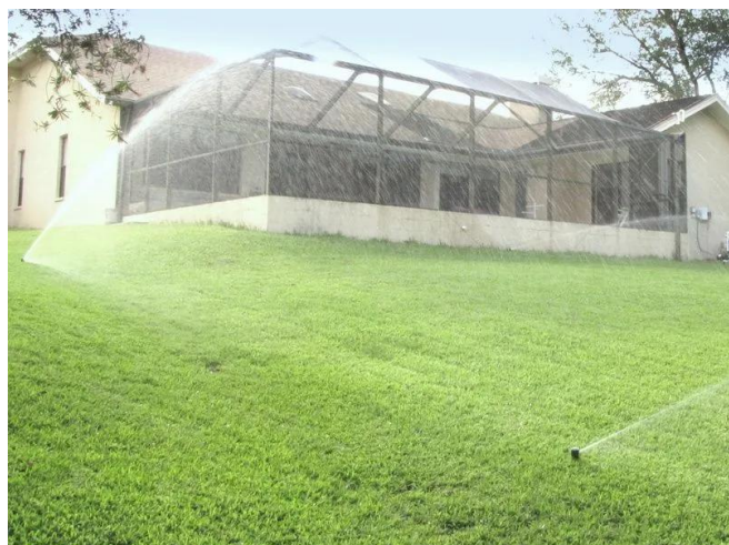
Figure 2. Gear-driven rotor irrigation heads. Credit: Bernard Cardenas, UF/IFAS
