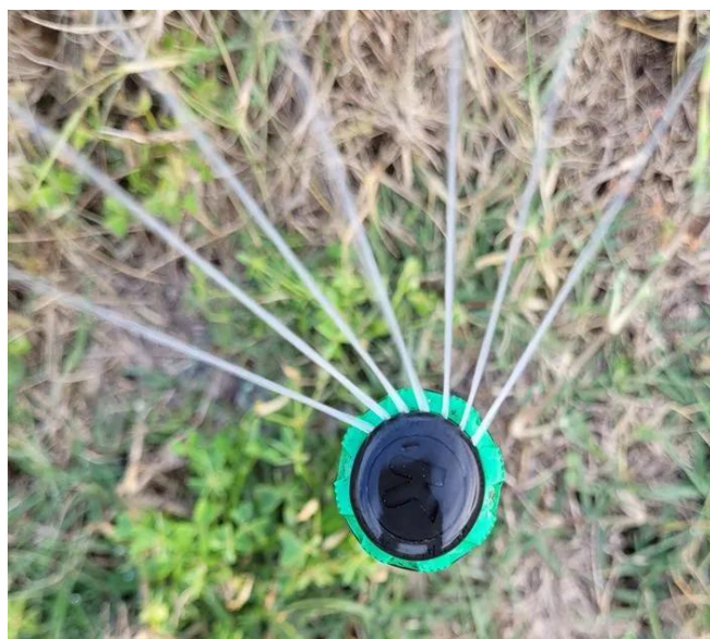
Figure 4. Standard head with a high-efficiency rotary nozzle. Credit: Bernard Cardenas, UF/IFAS
