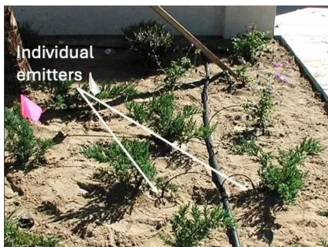
Figure 5. Individual drip emitters.
