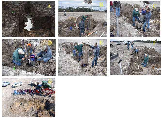
Figure 8. Installation of drainage lysimeter in UF/IFAS NFREC—Suwannee Valley, Live Oak, FL. A) Groundwater table visible. B) Inserting steel pipe to prevent soil from collapsing. C) Installing drainage lysimeter four feet below the soil surface. D) Drainage lysimeter within the steel pipe to keep the soil intact during lysimeter installation. E) Removal of the steel pipe after drainage lysimeter installation. F) Installing the PVC access pipes with the sledgehammer. Credit: Dr. Charles Barrett, UF/IFAS
