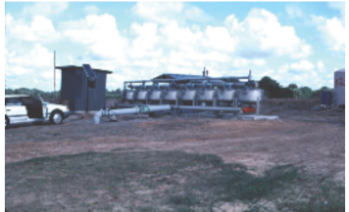
Figure 7. Media filters for filtering water used for drip irrigation of vegetables.
