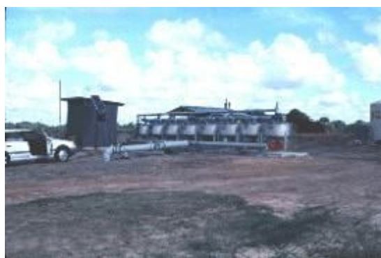
Figure 7. Media filters for filtering water used for drip irrigation of vegetables.
