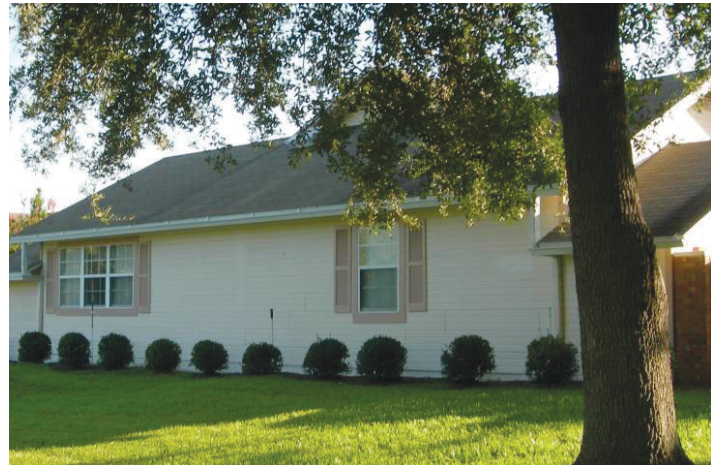
FIGURE 5. Shrubs along wall are overtrimmed.
