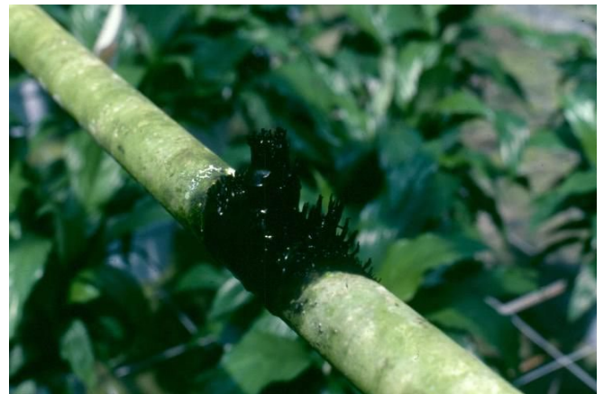
Figure 1. Algal growth is present on a nozzle that remains moist when the system is not operating. Credit: Tom Yeager, UF/IFAS
