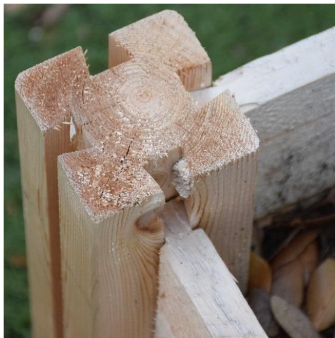
Figure 4. Example of corner post with grooves that allow 2" wood sides to slide in which makes it easy to construct and dismantle.
