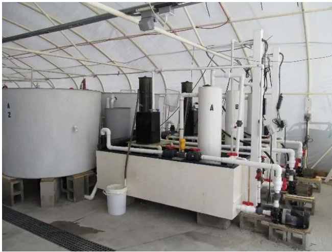
Figure 10. Recirculating system used in the culture of marine ornamental fish.
