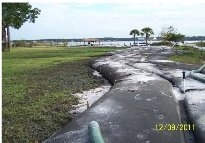
Figure 9. Large-scale muck removal using geofilter tube to dewater muck from Lake Down, FL. Credit: Sergio Duarte
