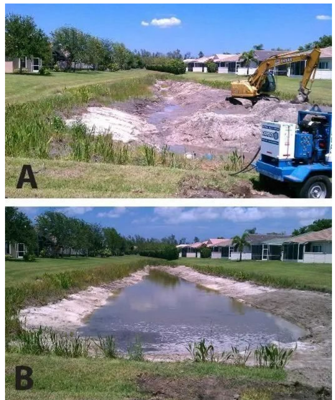
Figure 10. Picture of retention pond in Boynton Beach, Florida, before (a) and after (b) a small-scale dredging operations. Credit: Allstate Resource Management Inc.
