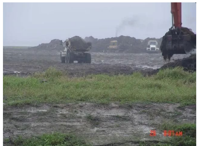
Figure 7. Heavy equipment moving muck during a lake restoration program for Lake Tohopekaliga, Osceola County, Florida.
