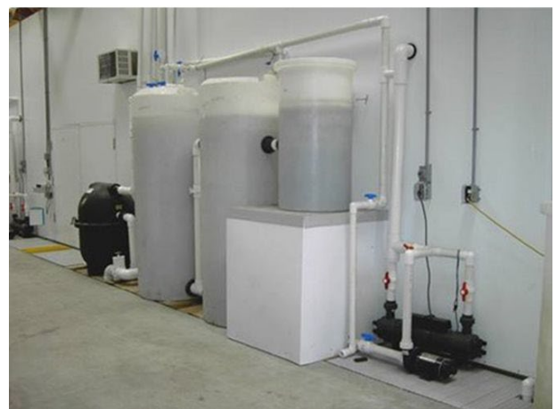
Figure 3. Broodstock holding tank design (28 m 3 ) and filtration components. Mote Marine Laboratory, Sarasota, Florida.
