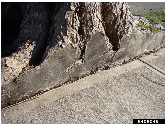
Figure 18. Construction is especially damaging to roots, such as these roots cut during sidewalk and curb repair.
