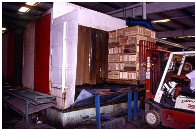
Figure 12. Cooling sweetcorn in a shower hydrocooler.
