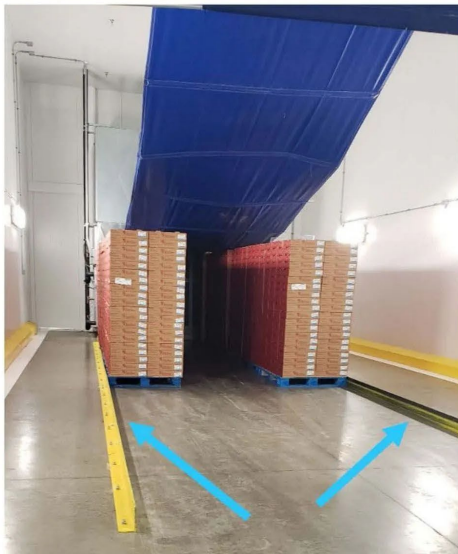
Figure 8-6. Side view at the front of a forced-air cooling tunnel showing: (top left) openings under blue foam pad and at the base of the white adjoining bin; and (top right) these openings blocked with corrugated sheets to improve cooling efficiency. In the bottom image, the fixed angle irons serve to align the pallets as well as block airflow underneath the pallets.
