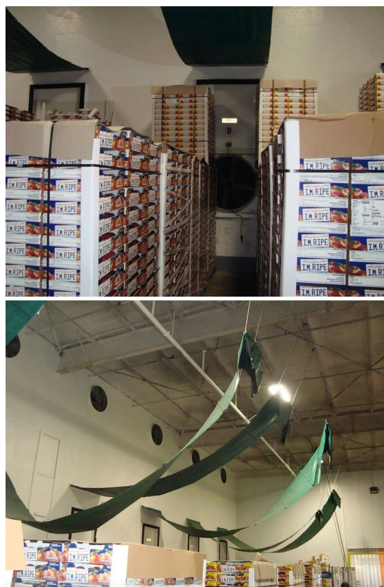
Figure 8-5. Forced-air cooling of peaches in palletized shipping cartons. The pallets have been aligned in rows on either side of fans set into the cold room wall to form the cooling tunnels, prior to lowering the tarps and turning on the fans to begin forced-air cooling.
