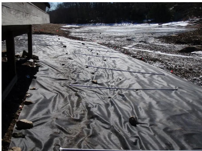
Figure 21. Benthic barrier (Aquascreen®) installed after a drawdown.
