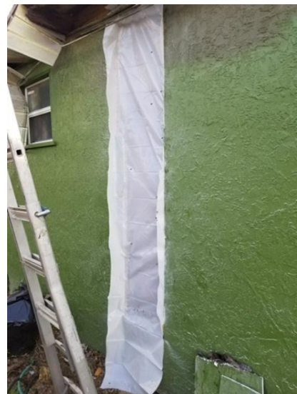
Figure 14. Unless you are a licensed and insured contractor, you should not attempt to repair a structure yourself. Flexible plastic sheeting can be used to provide a temporary seal.
