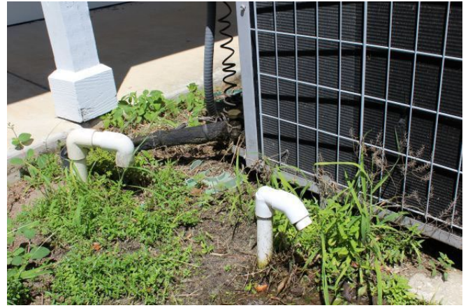
Figure 13. A/C lines should be directed away from the foundation.
