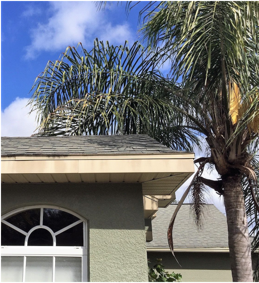
Figure 5. Palm leaves should be removed if hanging over a roof.
