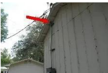
Figure 13. Opening around pipe.
