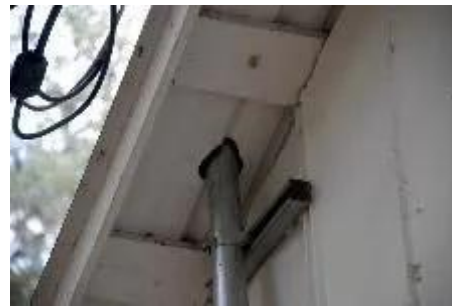
Figure 14. Opening around pipe.
