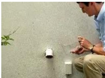
Figure 19. Placing screening over pipe.
