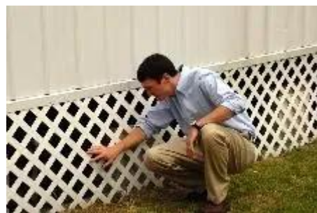
Figure 8. Inspecting under house.
