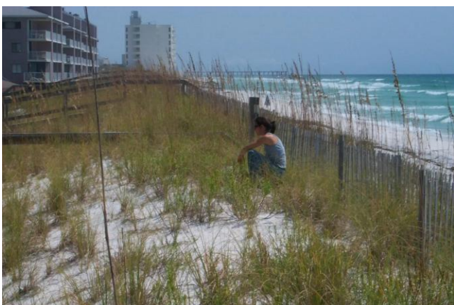
Figure 4. Constructed berm with sand fence located in front of coastal development and planted with a mixture of sea oats ( Uniola paniculata ) and bitter panicgrass ( Panicum amarum ) along Navarre Beach, Santa Rosa Island.
