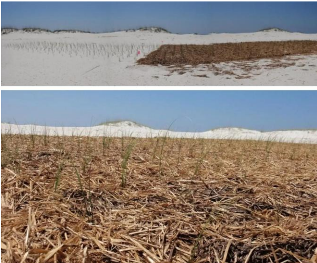
Figure 23. Foredune restoration site of sea oats ( Uniola paniculata ) planted approximately 12 in apart, the right half with an 8-inch layer of wheat straw two weeks after planting to serve as an artificial wrack. Below, the close-up view.
