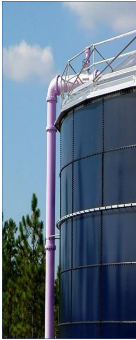
Figure 1. Reclaimed water reuse storage tank. Credit: Shanin Speas, FDEP
