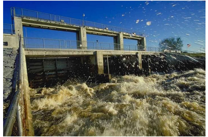
Figure 11. Water management structure releasing water (SFWMD).
