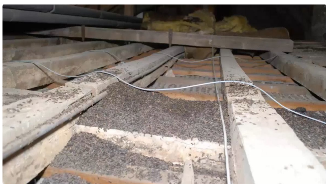
Figure 3. Large accumulation of bat guano indicating presence of a bat colony.
