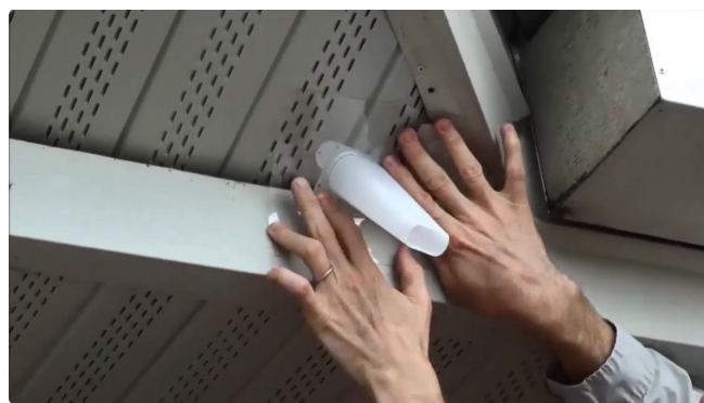
Figure 4. Installation of a temporary one-way exclusion tube over the exit/entry point.
