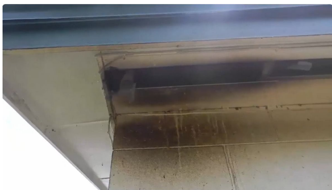
Figure 2. Staining is evidence of bats using an entry/exit point along a roofline.
