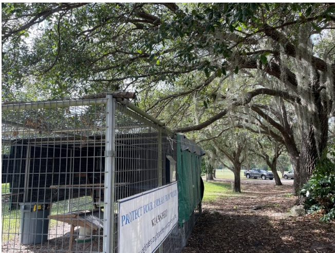
Figure 4. Trees and branches over a coop provide shade but can also be a hazard during storms.
